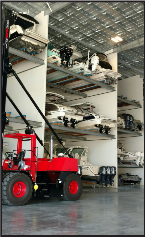
Concrete tilt wall construction and custom metal roof, steel bunk beams supported by concrete wing walls.
