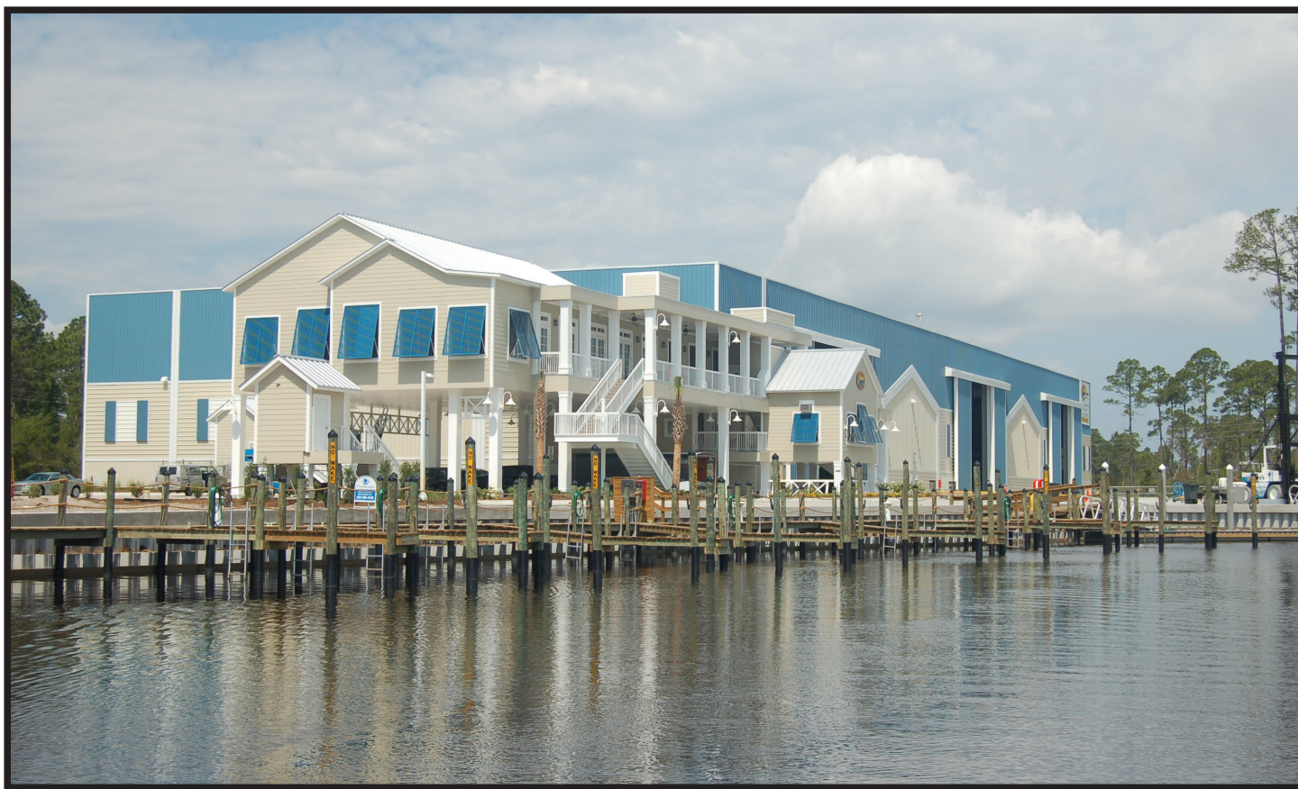
A rack-supported metal building with a capacity for 300 boats that are 25'-40' LOA. Also features a clubhouse, offices adjoined to building, and 2 fork lifts.
