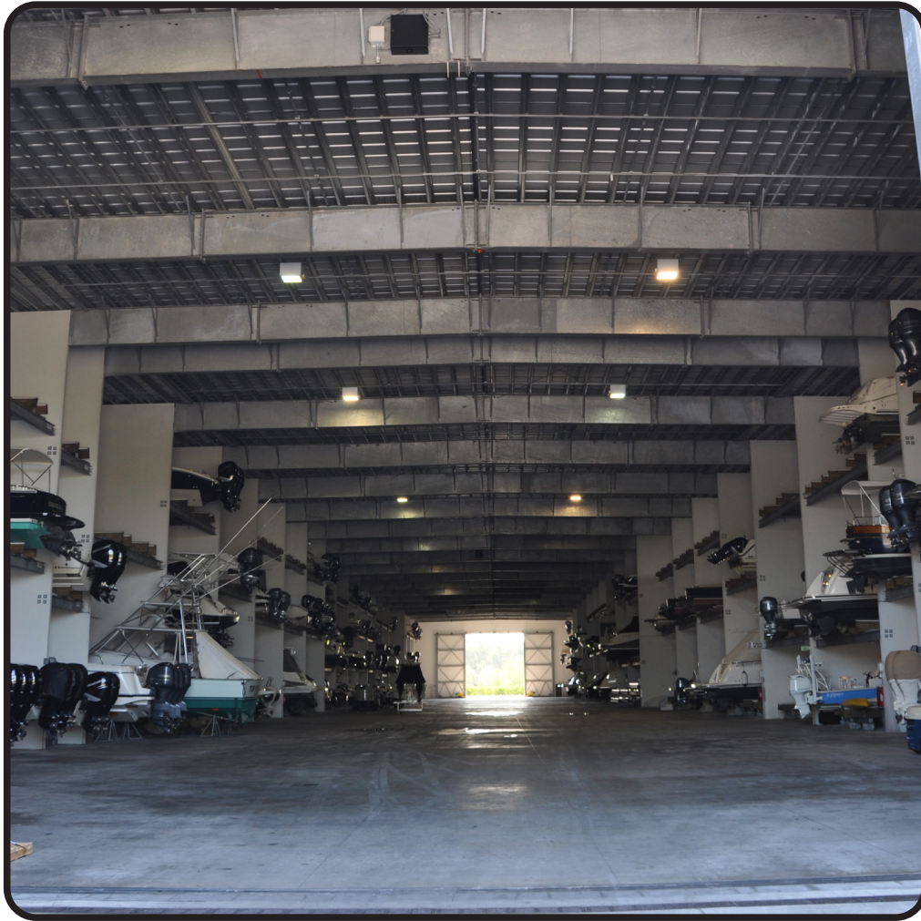
Reinforced concrete wing walls support racks and roof.
