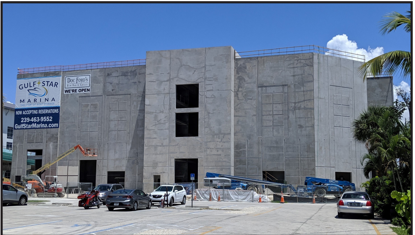
Street side view of the concrete tilt wall Dry Storage building in final stages of construction.
