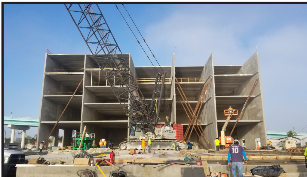
Boat storage bays with concrete wing walls and bunks under construction.
