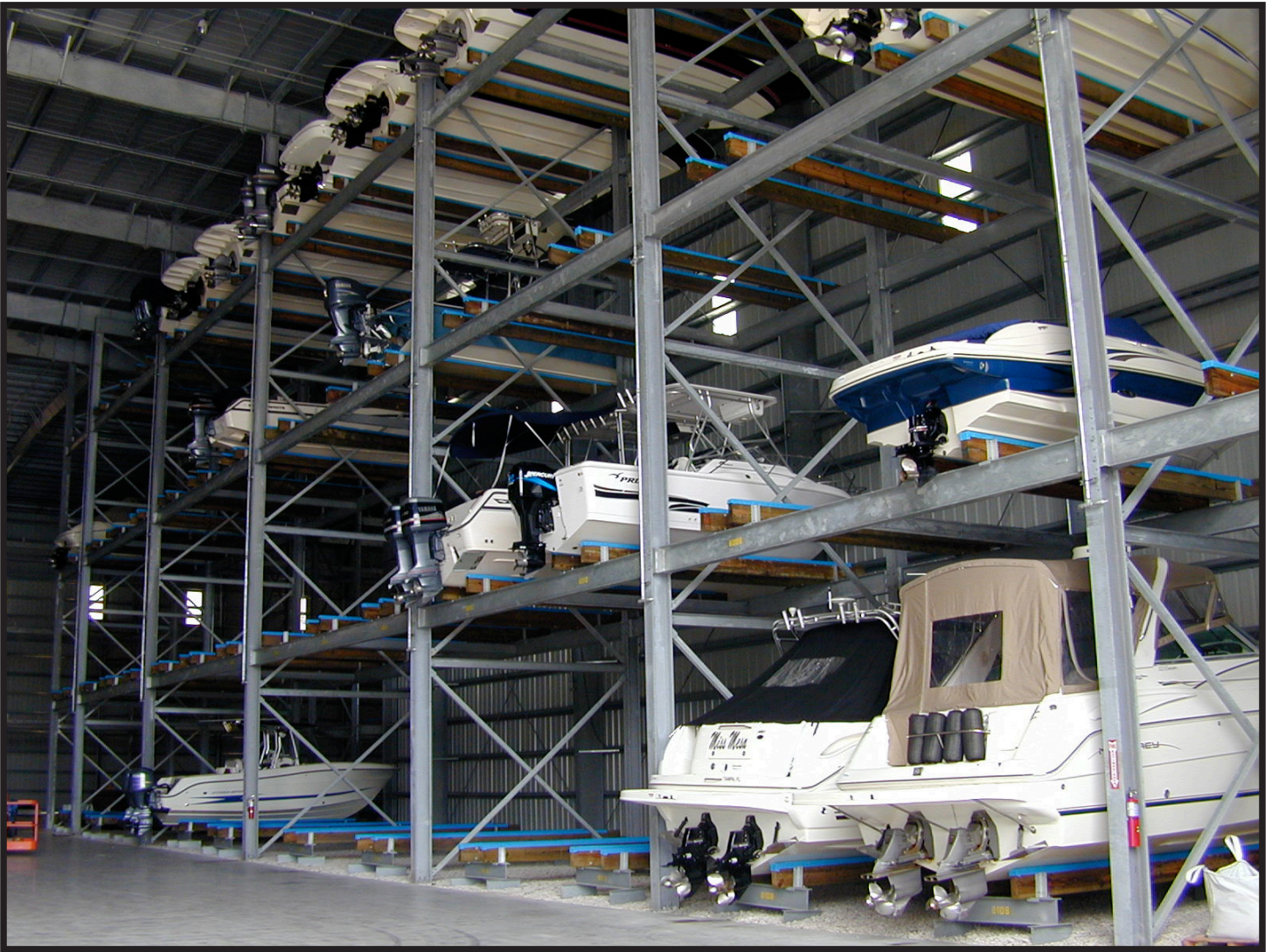
35' LOA boat racks at Nautico. Blue bunk coverings for greater visibility to assist fork lift operator.
