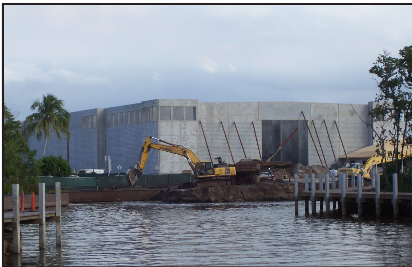
Hamilton Harbour tilt wall concrete construction.
