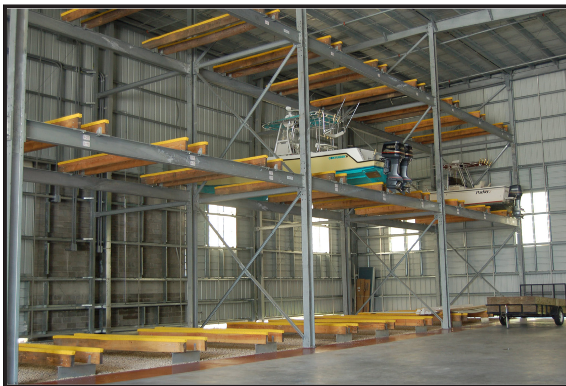
35' LOA bay section. Yellow bunk coverings for greater visibility to assist fork lift operator.
