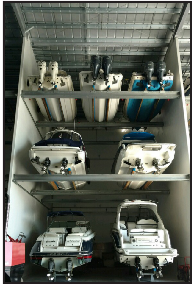
Concrete tilt wall construction and custom metal roof, steel bunk beams supported by concrete wing walls.
