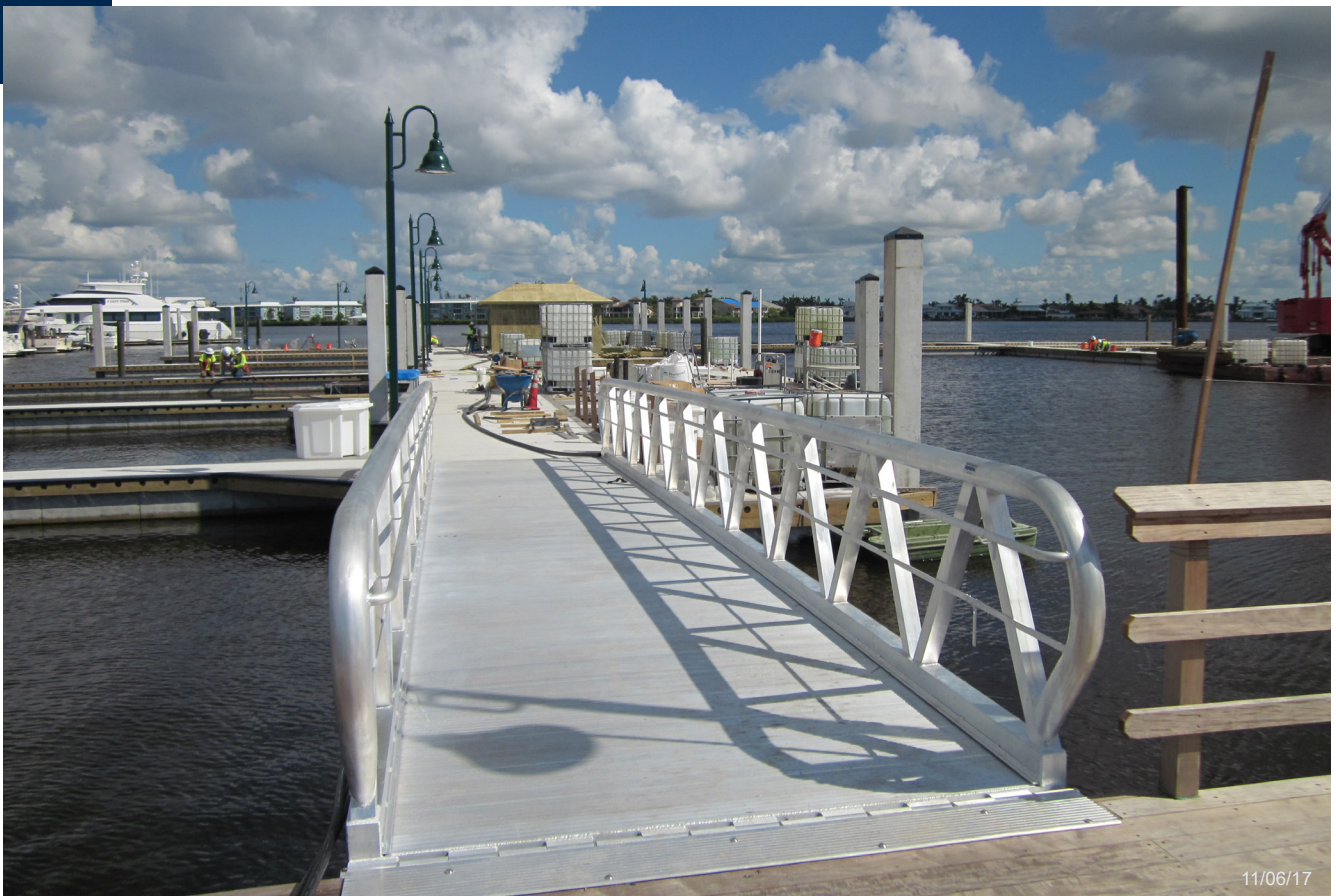
Aluminum gangway in place and secure between fixed access dock and floating dock.
