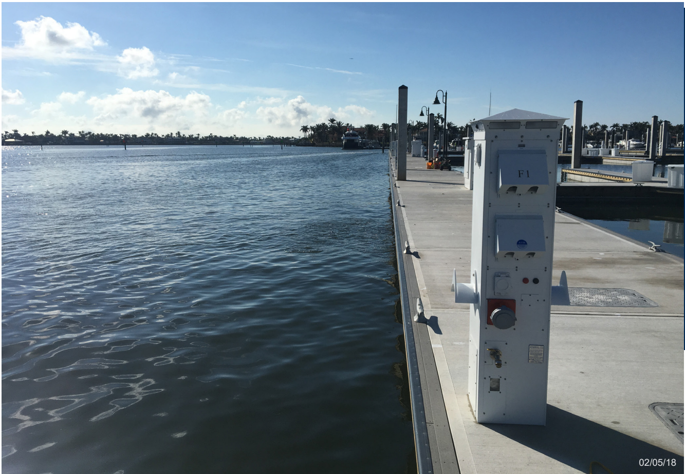
View down main wharf on Naples Bay, with shore power electric pedestal in place and ready for boats.
