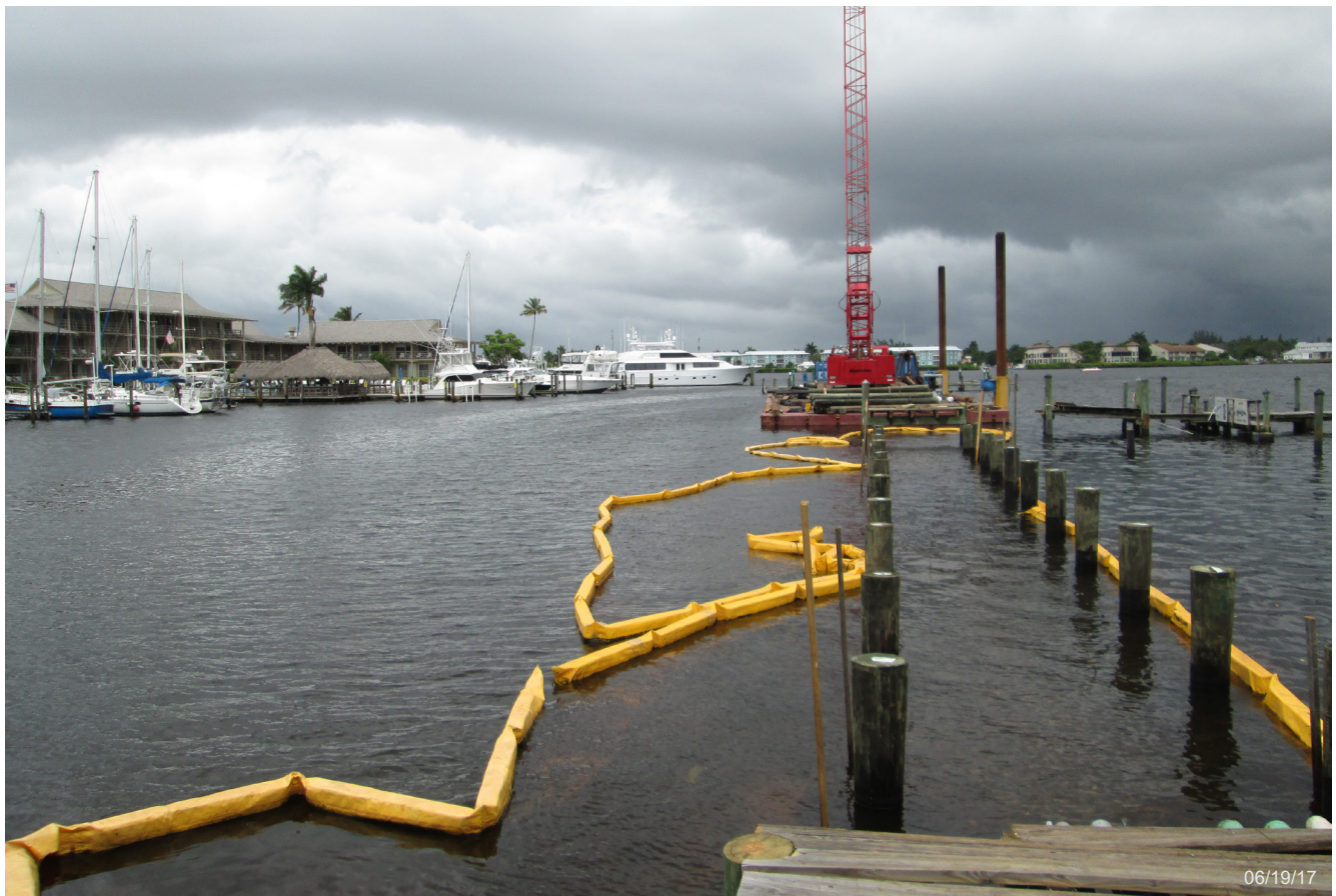
New pilings installed for the fixed access dock.
