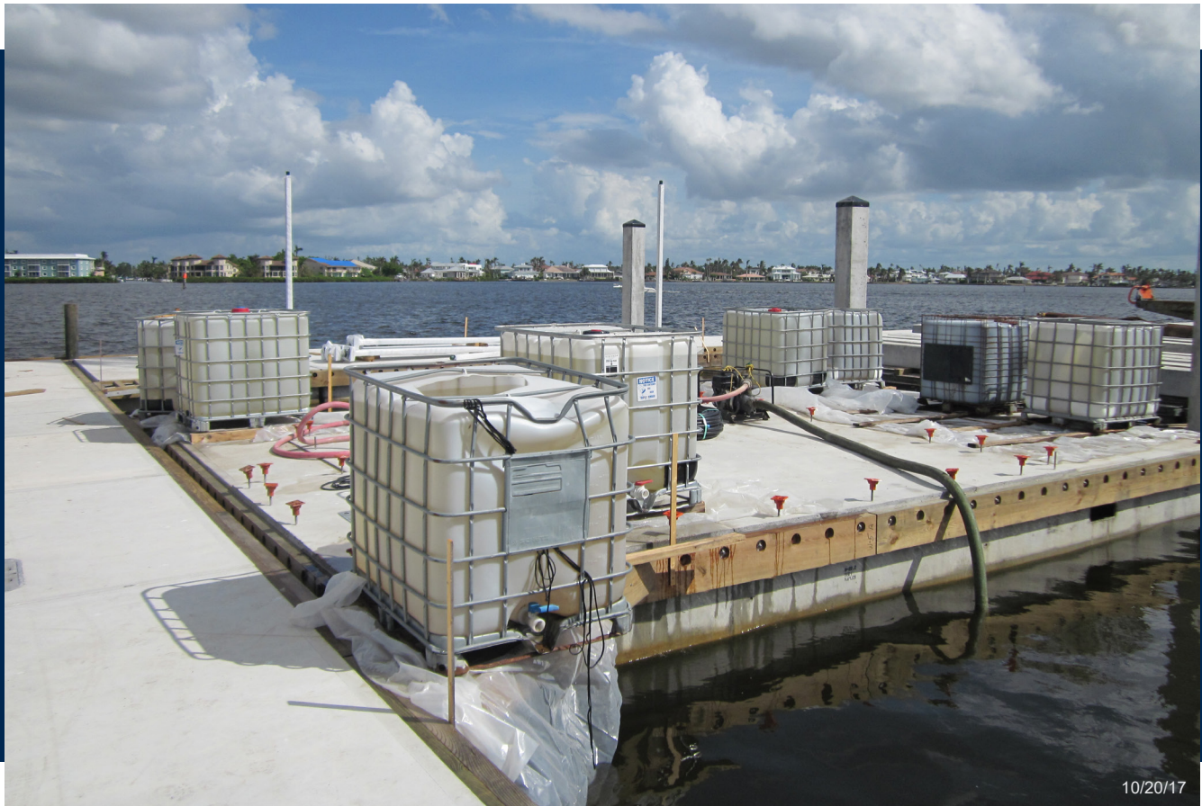
Building float in place with water tank ballasts to compensate for the building to come.
