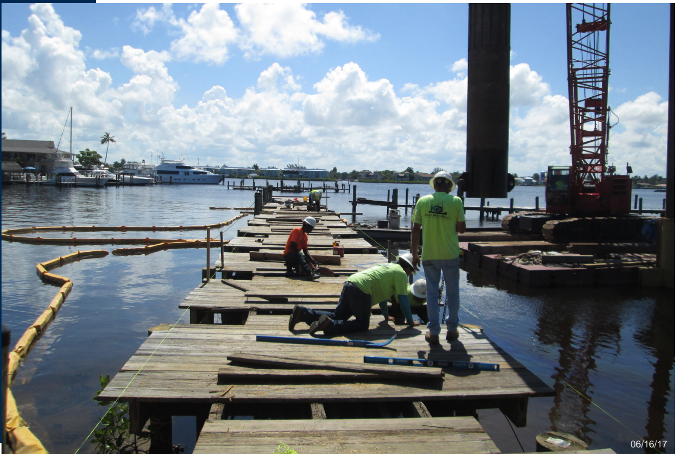
Decking is removed from the old fixed dock.
