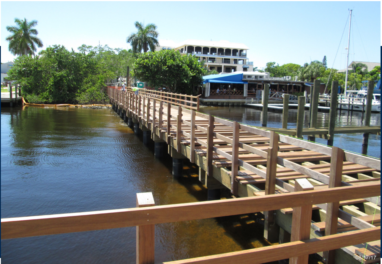
Framing for the fixed access dock from shore.
