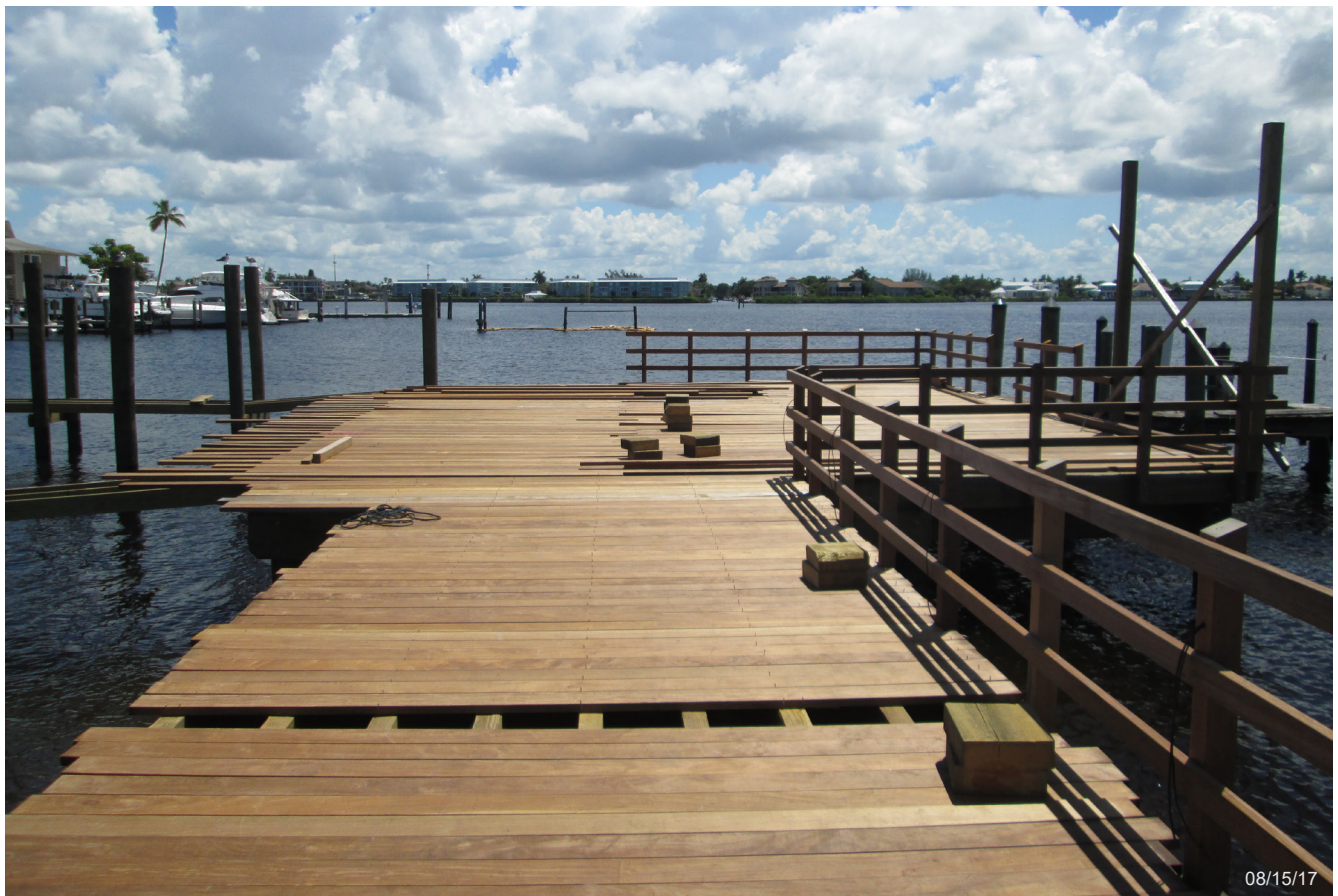
IPE decking going on the end platform of the fixed access dock.
