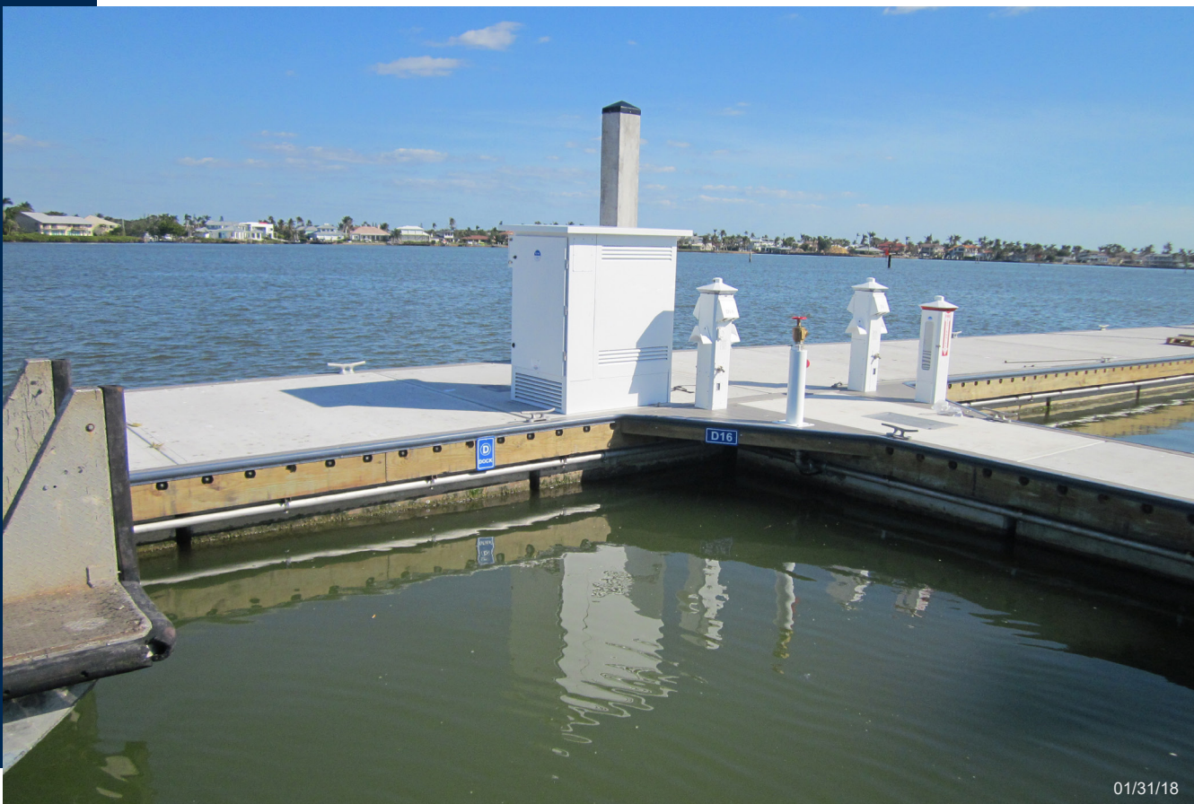
Large electrical transformer on bay front wharf with smaller pedestals for boat plug in shore power.
