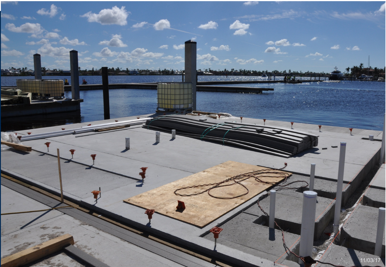
Concrete float for Restroom Complex in place and ready for building structure.
