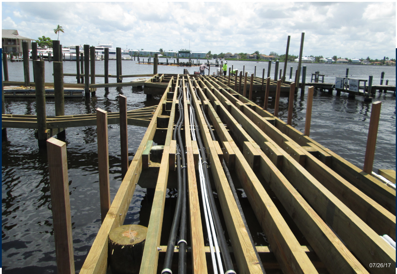
Framing and utility conduits in place.
