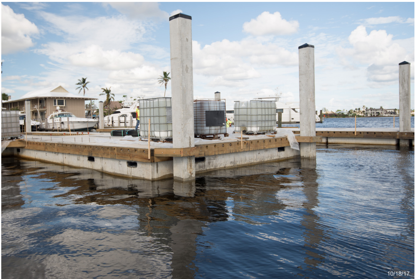
Concrete float for the Dockmaster's Office in place with concrete control piles.
