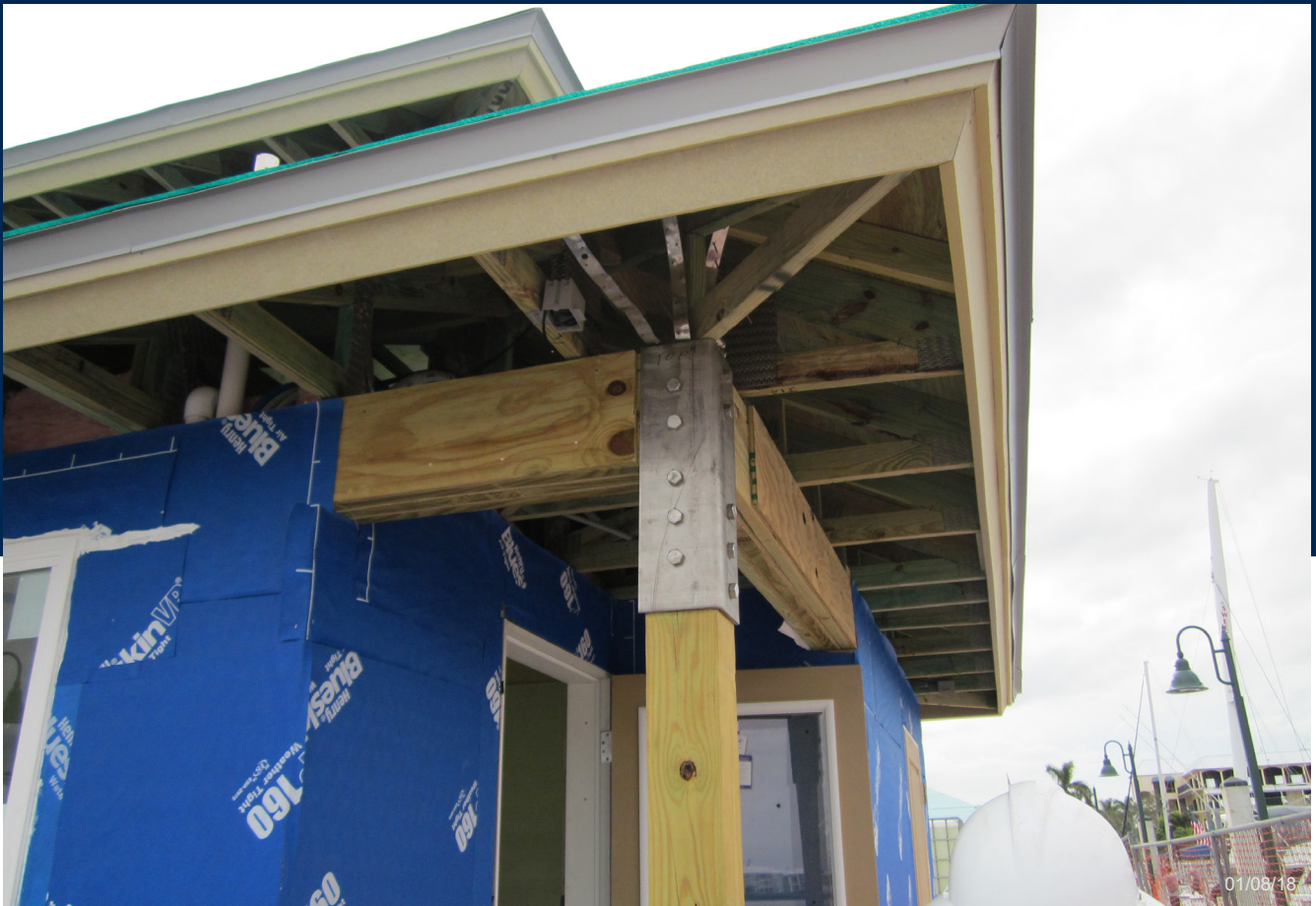
Structural attachment, built to withstand 170mph winds.
