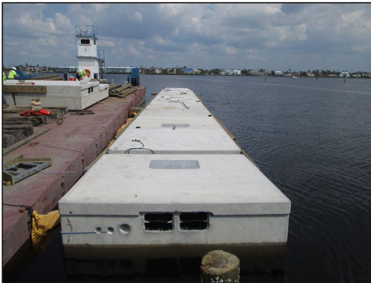
Concrete floating dock alongside barge on site, being moved into position. Note chases inside of dock.
