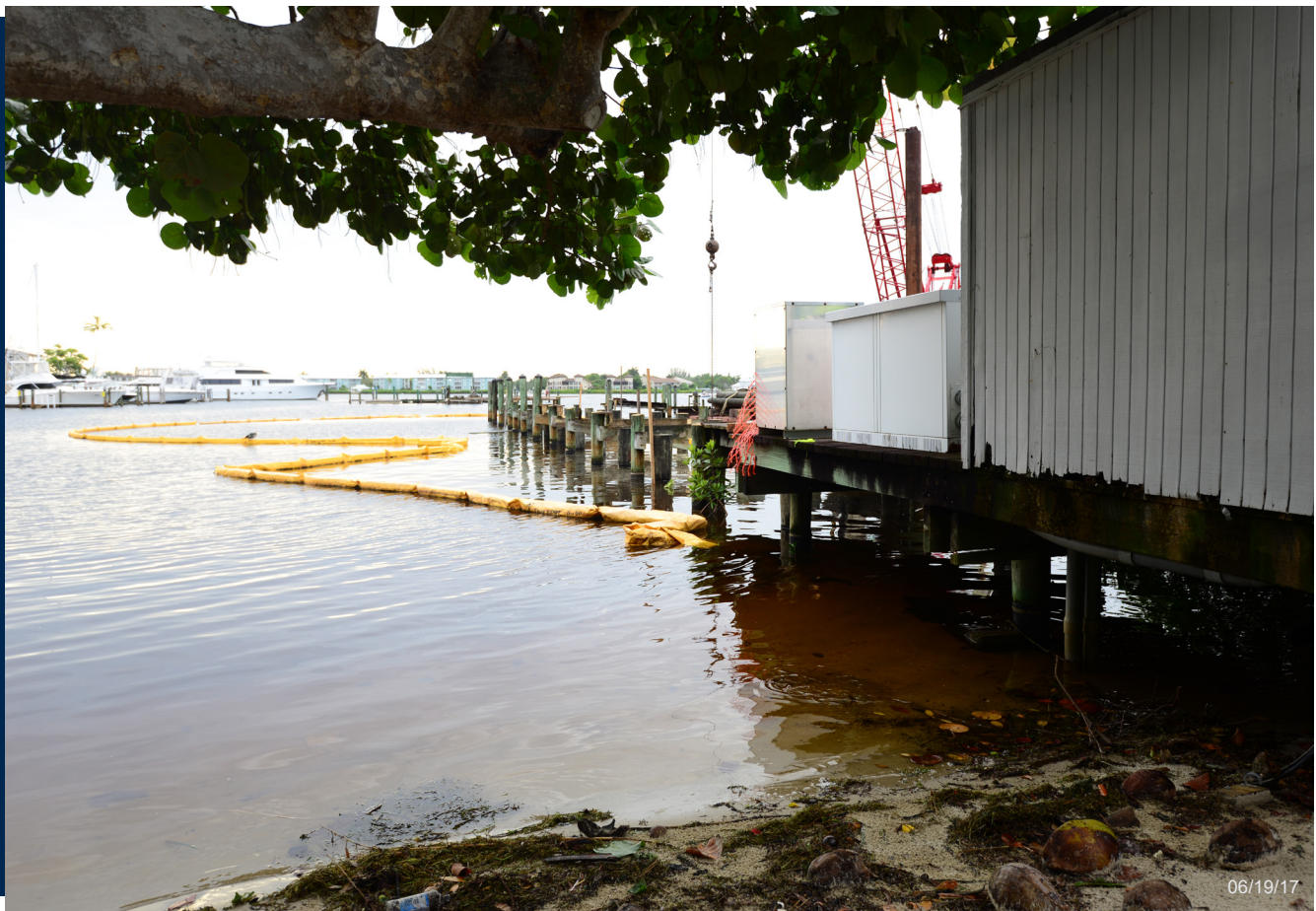
Yellow turbidity curtain keeps debris contained in demolition area.
