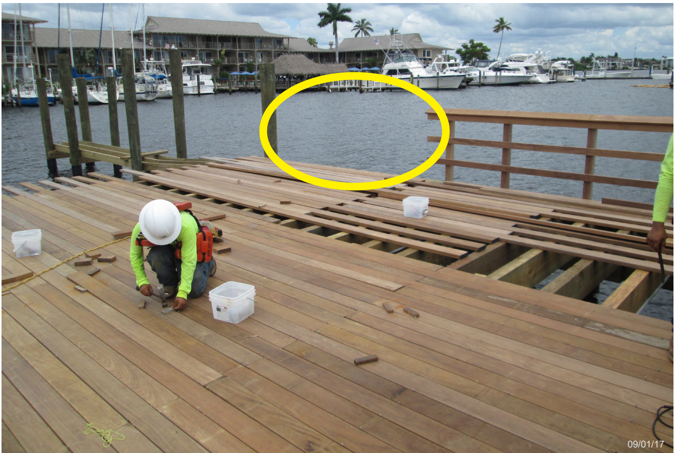
Finishing the end platform, note space in railing (circled) ready for gangway attachment to the concrete dock.
