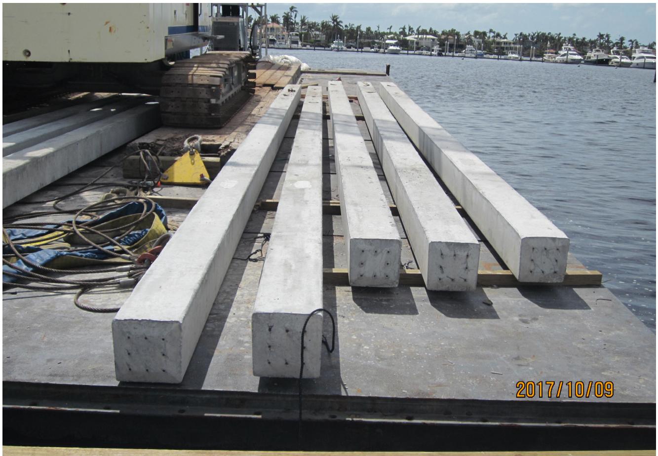
Concrete control piles arrive that will be used to keep the floating docks in place.
