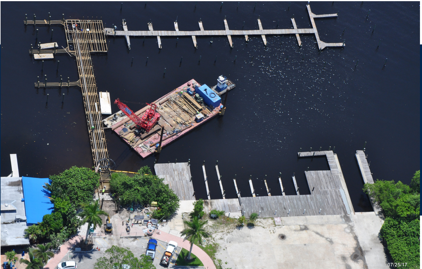
Framing for fixed access dock being completed.
