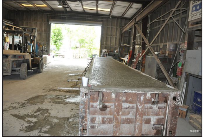
Concrete floating dock in form curing.
