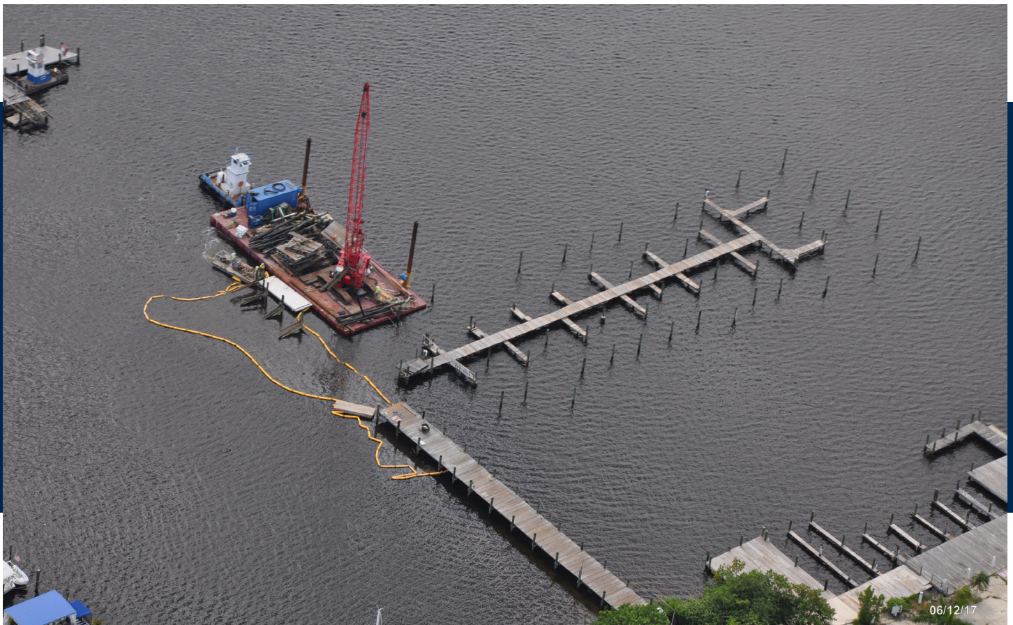
Demolition of the old wood docks in progress.
