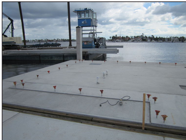
Concrete float for City Dock's Restroom Complex is put in place during construction. One section of dock ready to be joined with the next to create the base floor for vertical construction.
