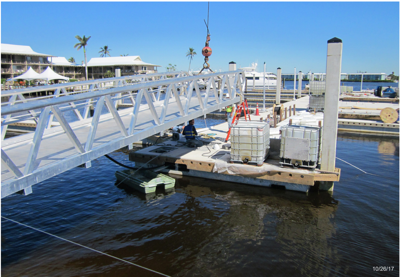
Aluminum gangway to floating docks being installed.
