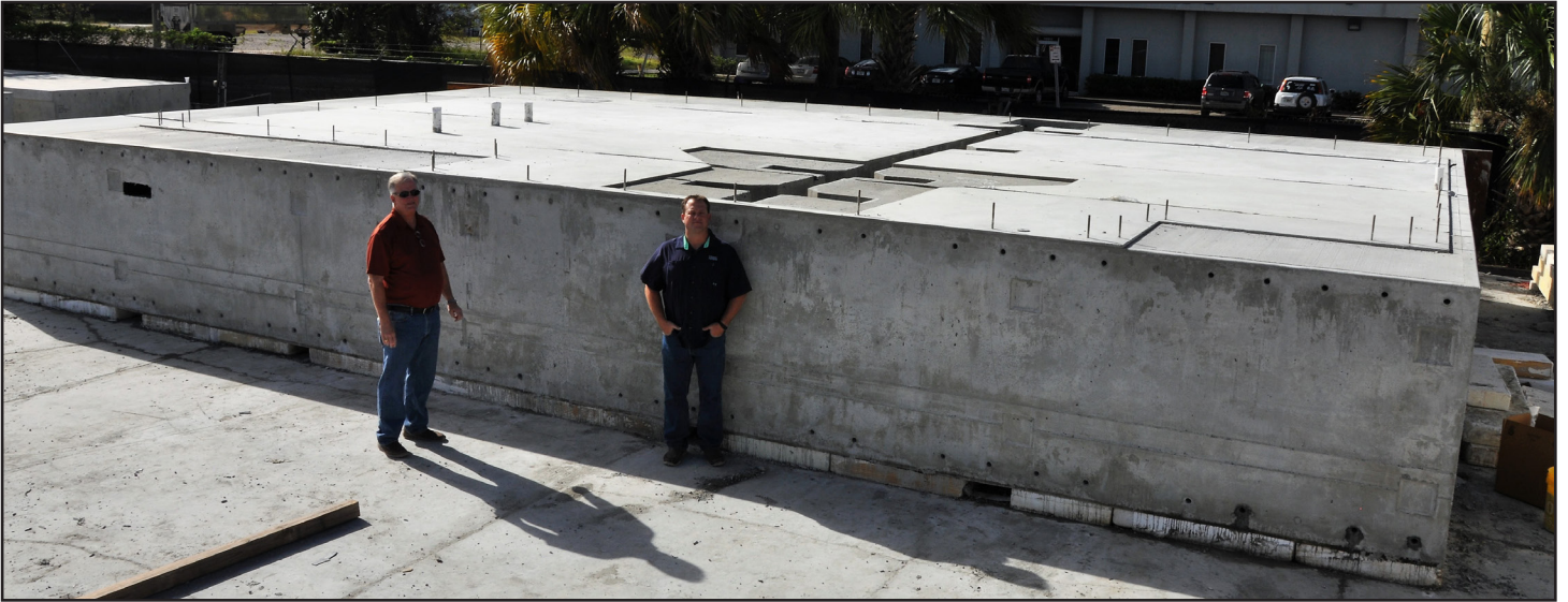
Massive concrete floats for City Dock's Restroom Complex in Bellingham's Jacksonville yard awaiting transport.
