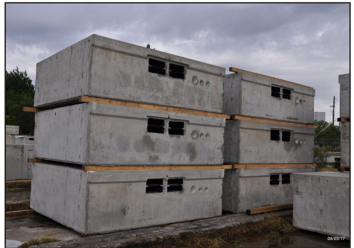
Floats stacked and curing, utility "chase" (special openings where the electric lines run through the concrete) shown on sides.
