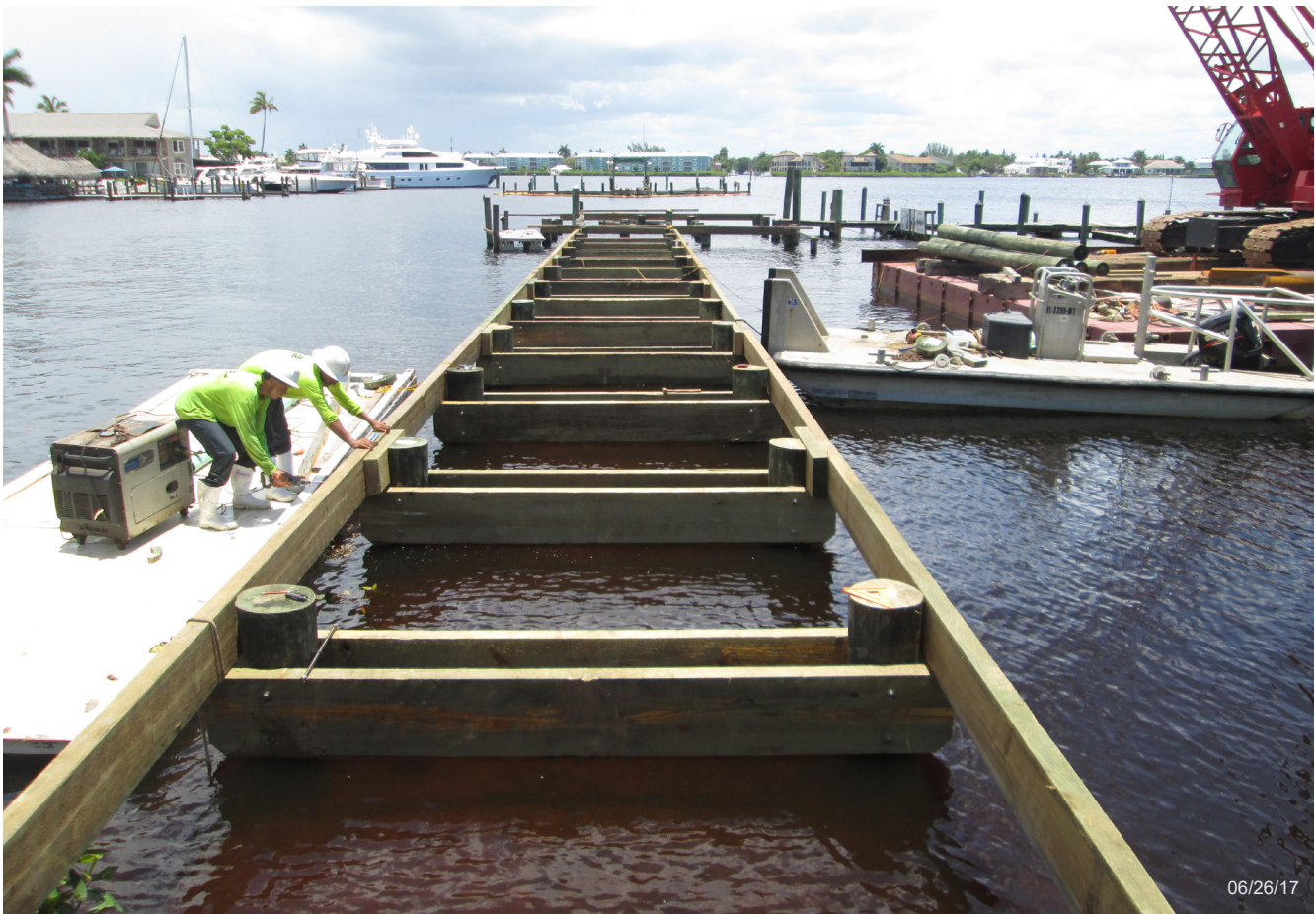
Above and below: Framing going in for new dock.
