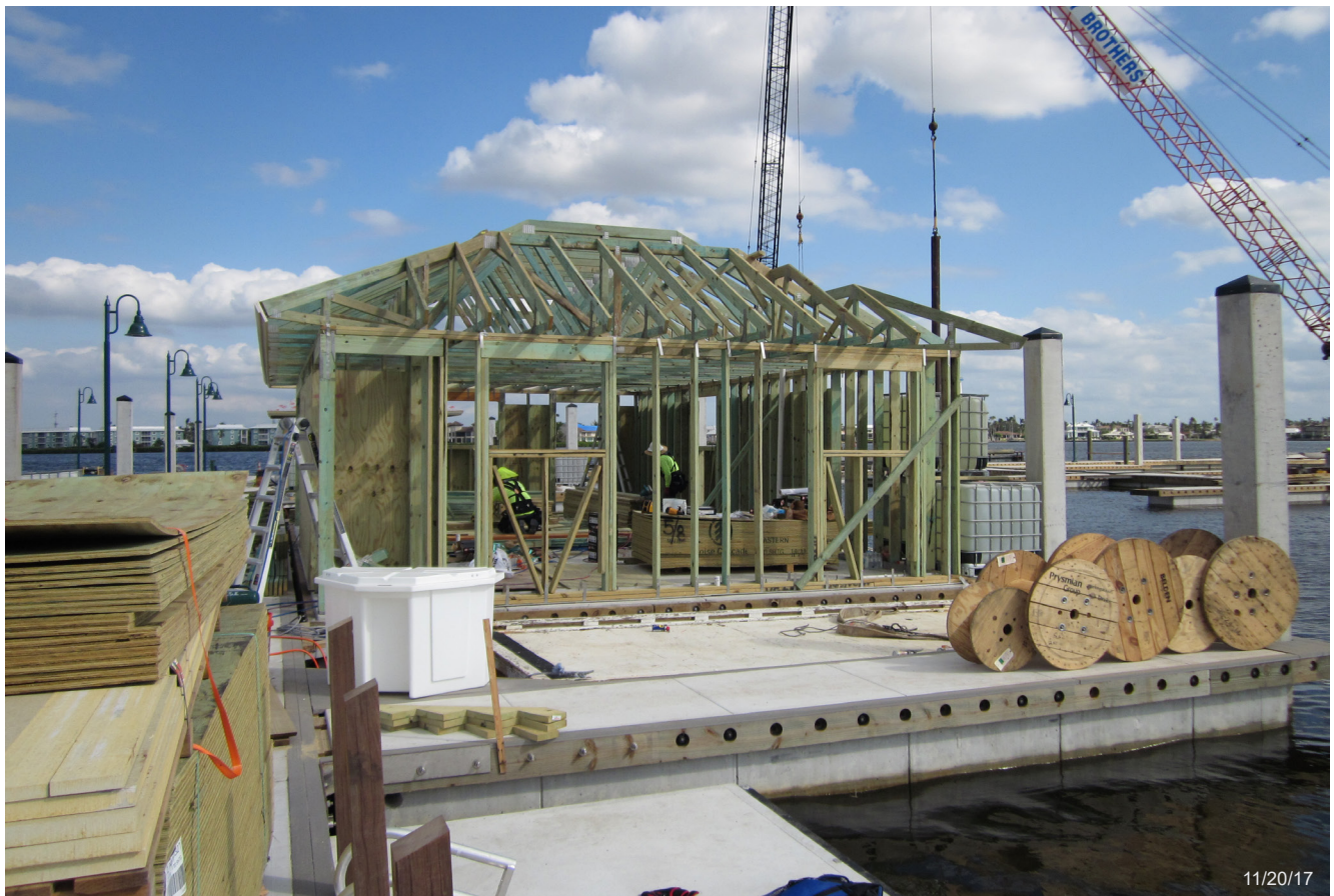
Framing for the Restroom Complex.
