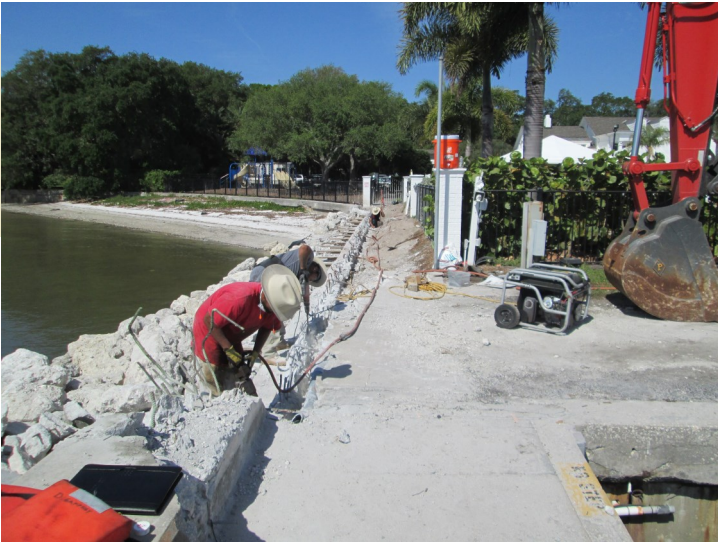
South seawall cap removal.
