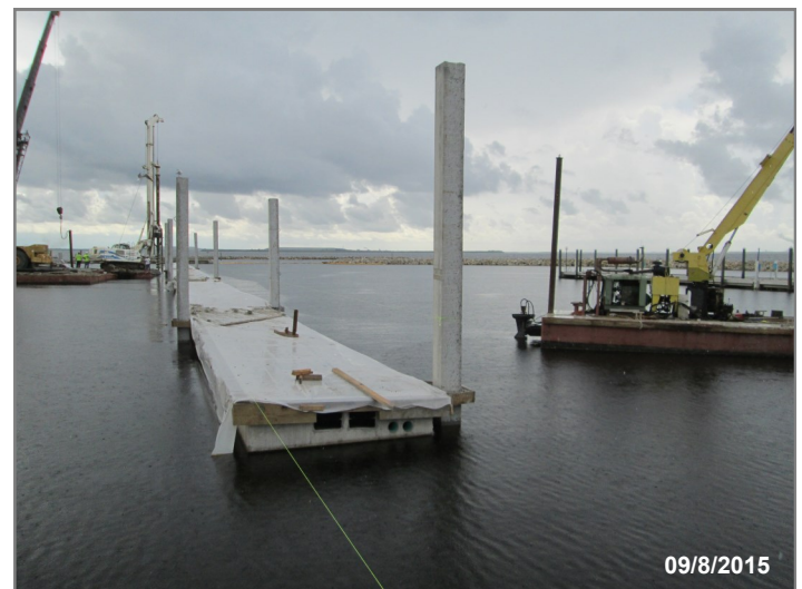
New floating system under construction for B & C Dock.
