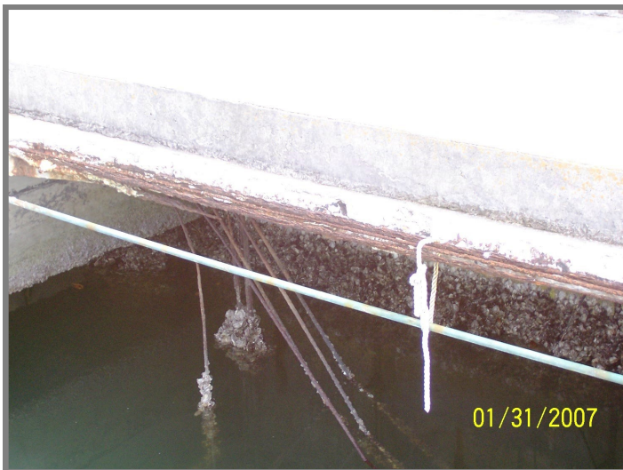
Existing seawall showing reinforcement steel.
