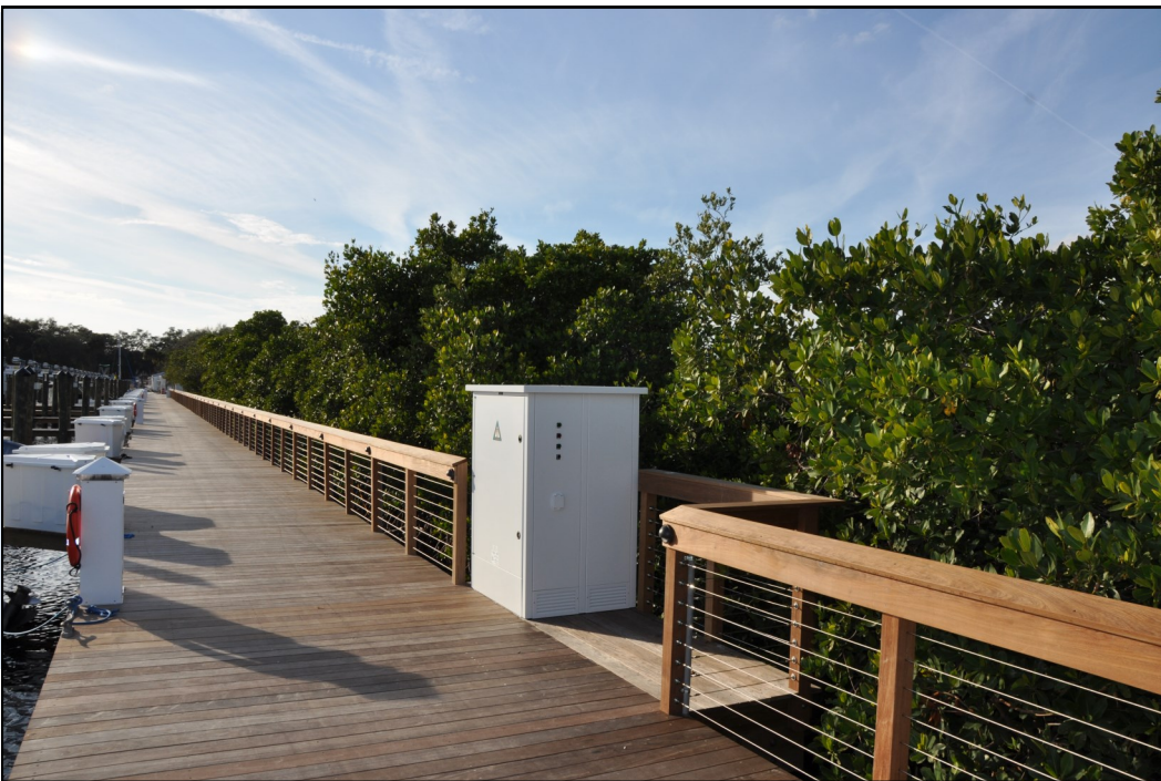
A Dock with IPE deck and railing finished in stainless cables.
