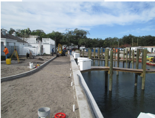
Marina walkway ready for concrete pad and walkway pavers.
