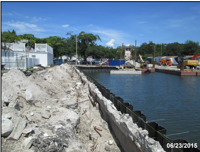
New seawall being installed in front of the old seawall.
