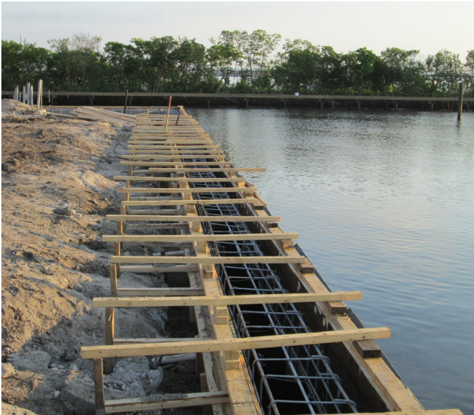
Seawall cap ready for concrete placement.
