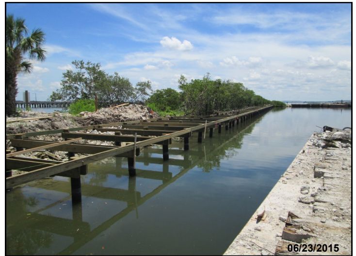
Framing in place for the new A Dock.
