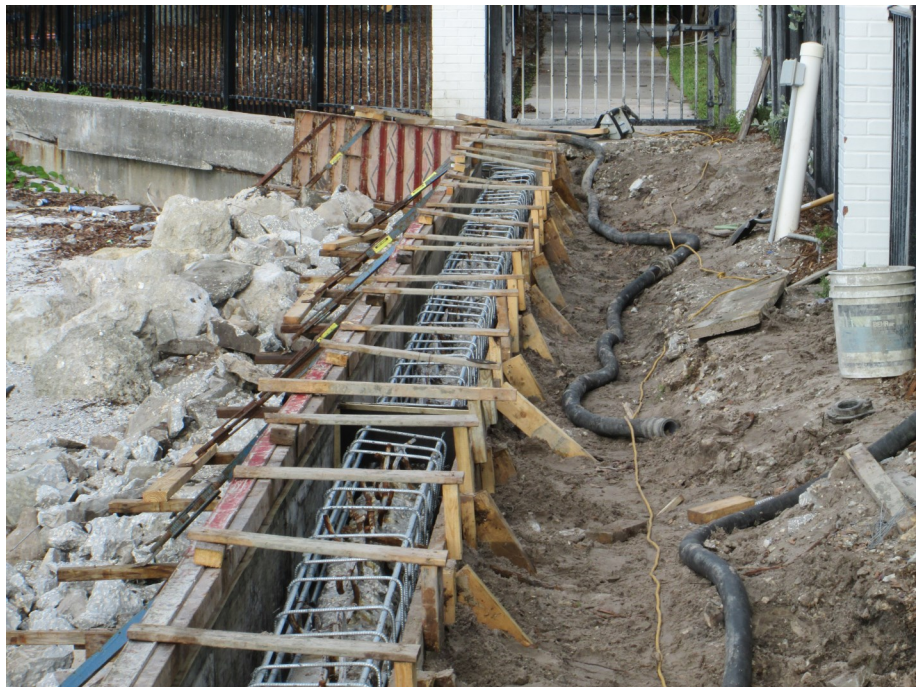
Forming the new seawall cap.
