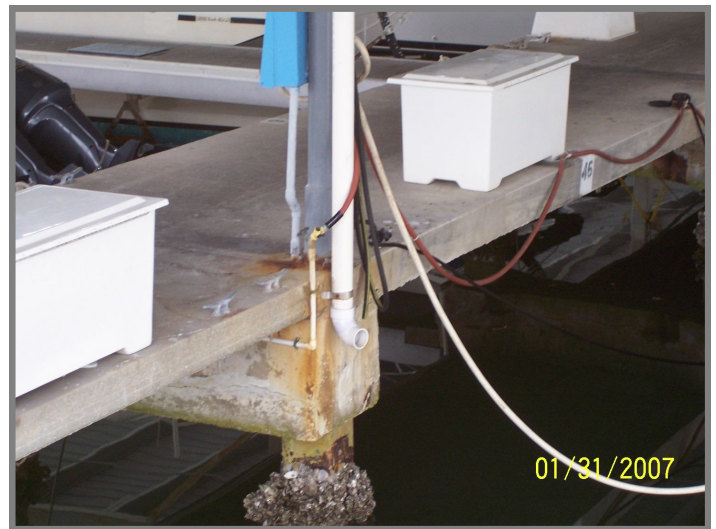
Concrete support cap, cracked and deteriorating.
