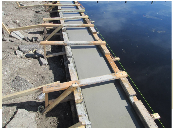
Freshly poured concrete cap.
