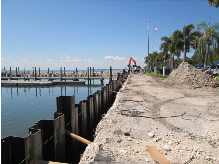
Seawall panel installation seaward of the old wall.
