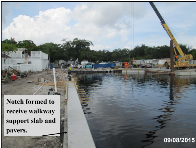
Concrete seawall cap during construction.
