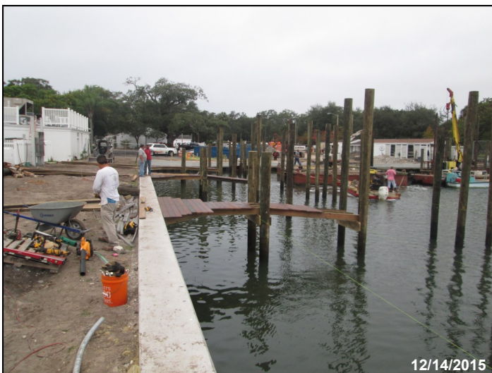
Finger piers under construction in front of new seawall.
