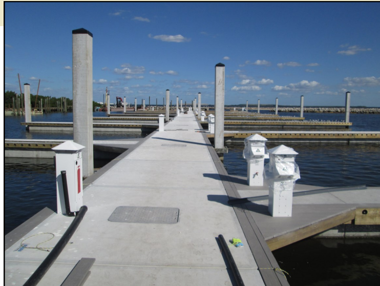
Power pedestals and fire cabinets in position.
