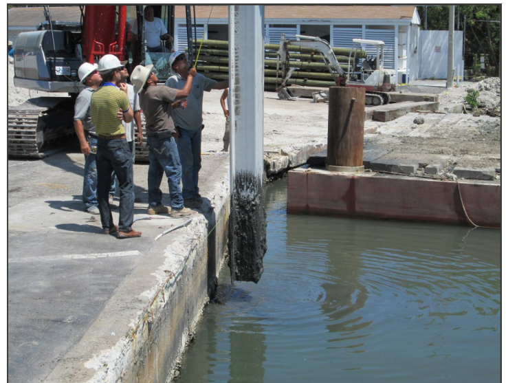
Testing seawall penetration with a sacrificial panel.
