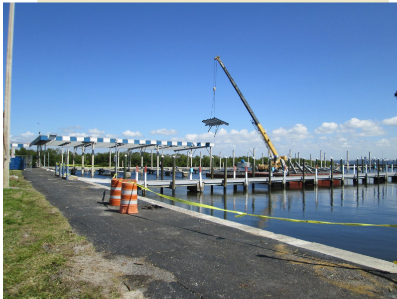
Roof dismantled and loaded onto barges.
