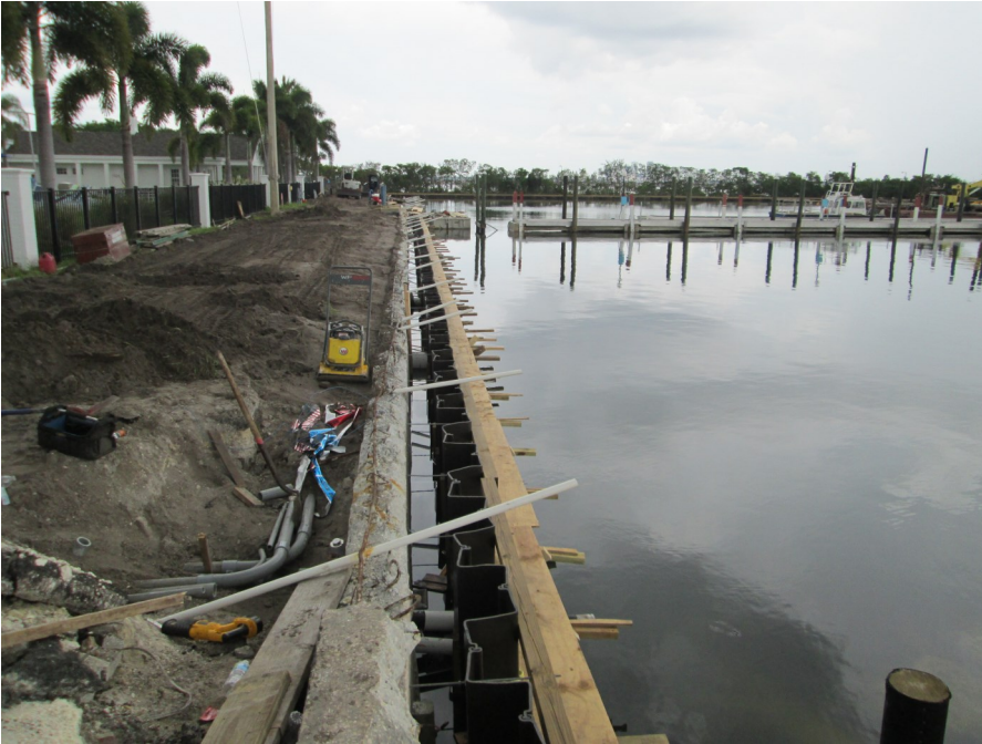
New tie back rods being placed which will tie into the concrete cap to support the wall.
