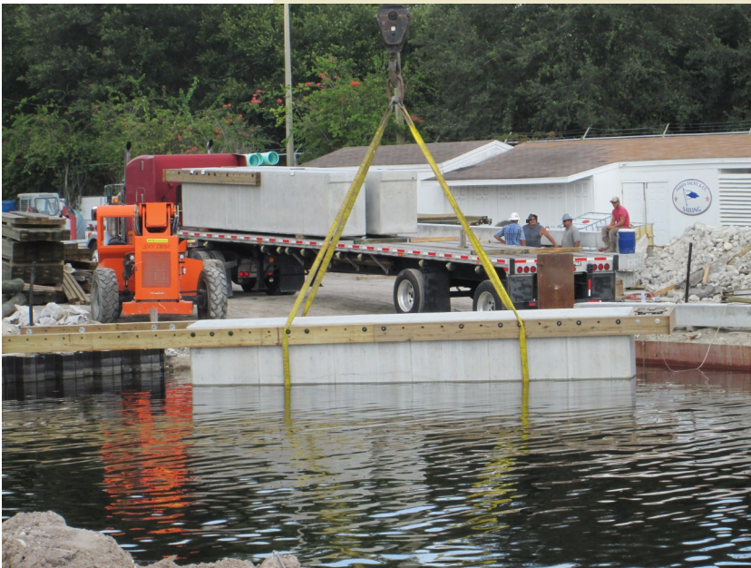
Concrete floating docks being unloaded and "splashed."
