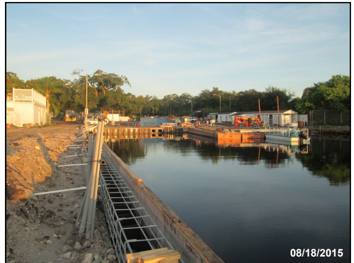
Seawall cap being formed for concrete placement.
