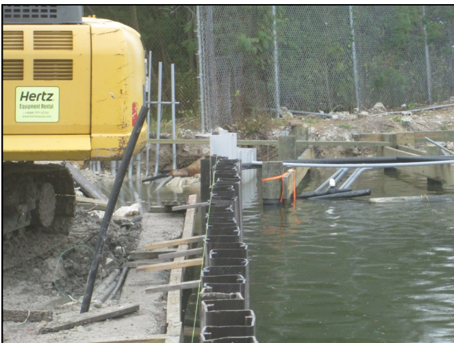
Final seawall panels installed adjacent to A Dock.
