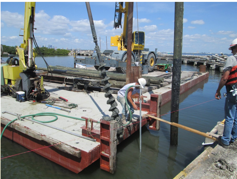
Piling installation.
