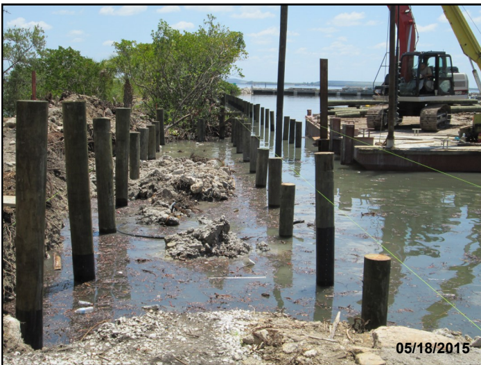
Pile installation.
