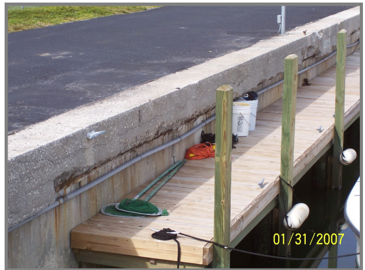
Deteriorated seawall showing cracks and exposed rebar.
