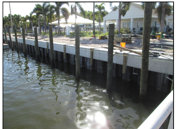
Piling complete for fixed dock along seawall face.
