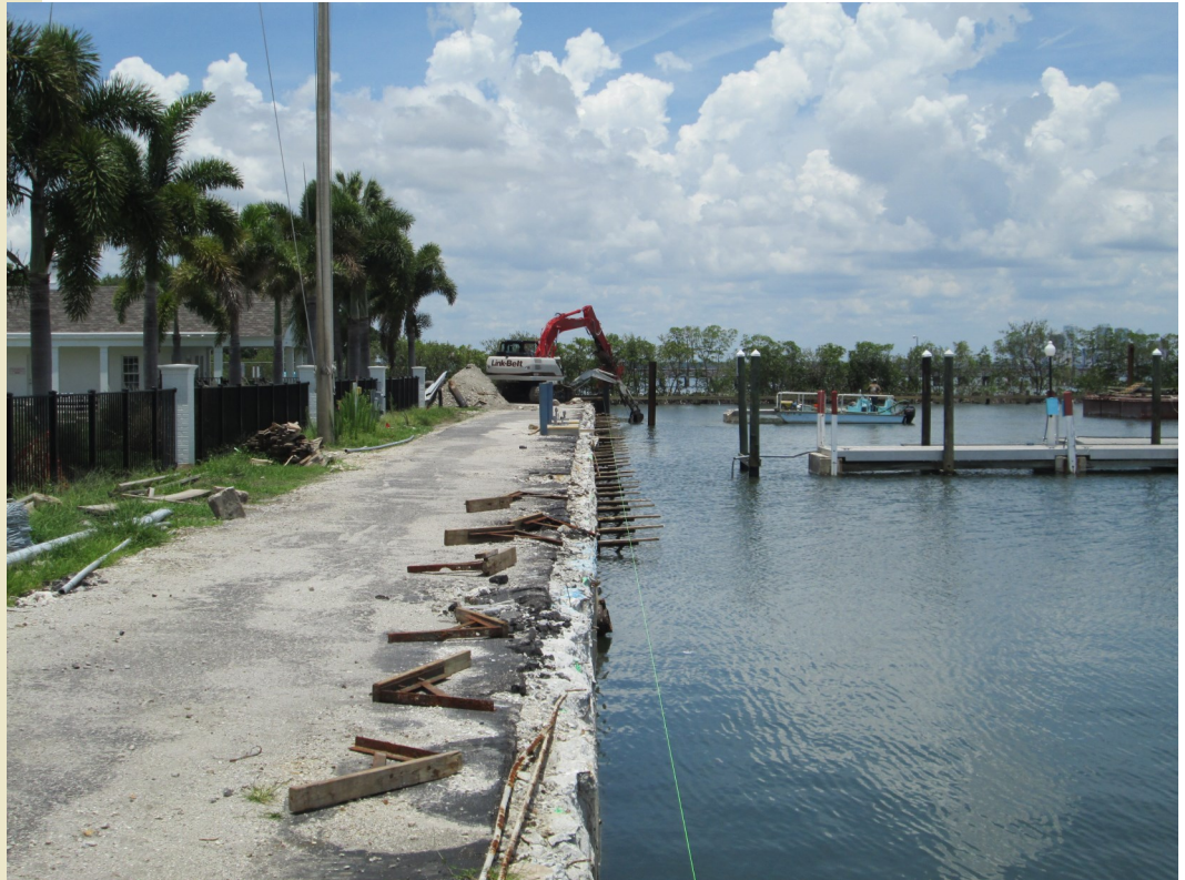
Seawall cap removal complete.
