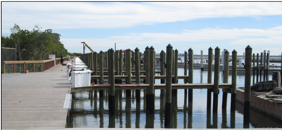
New piling supported structure with IPE decking.
