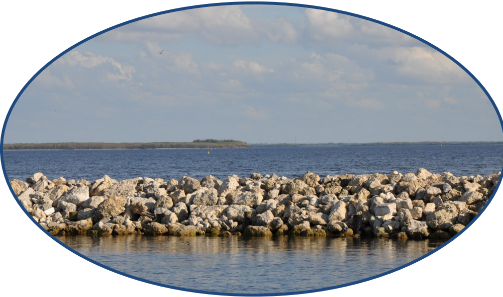
The rock breakwater was designed to be left intact on the seaward side to maintain its strength. The old concrete decks and seawall cap on the inside were broken up and entombed in new rock to create a clean, natural look.
