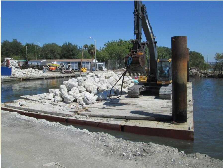
Loading breakwater rock on a barge from shore.
