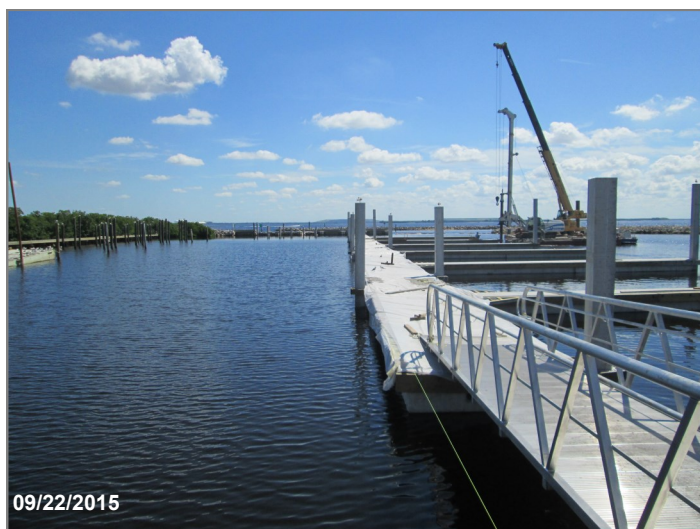
Concrete control piles being installed.
