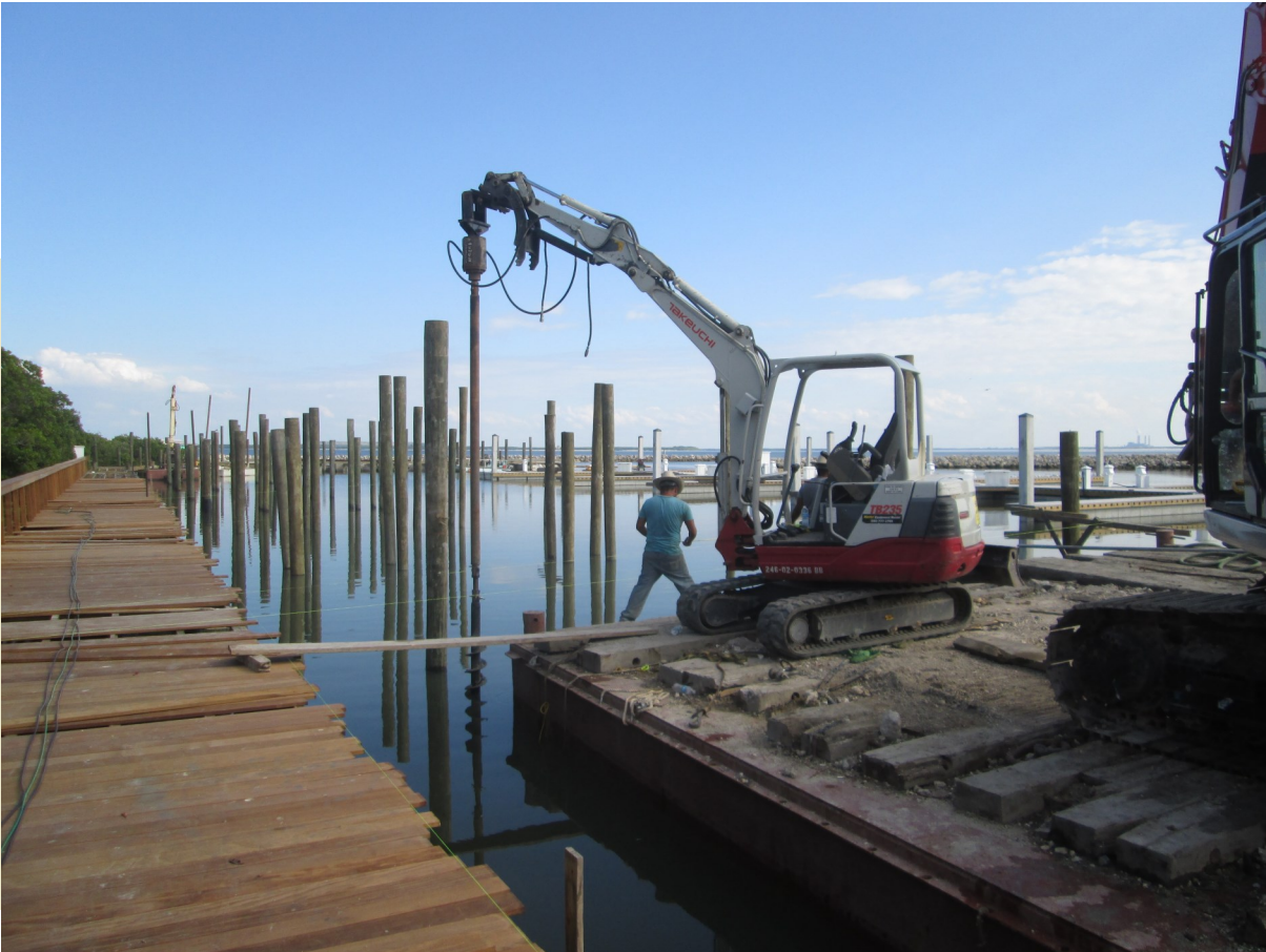
Finger pier construction.
