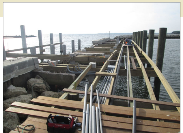
Utility conduits being installed below deck.
