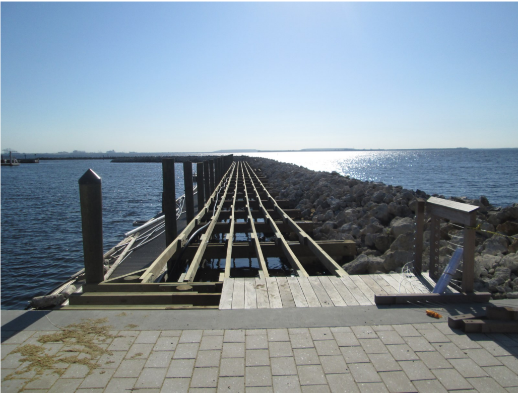
Dock framing in progress on F Dock.
