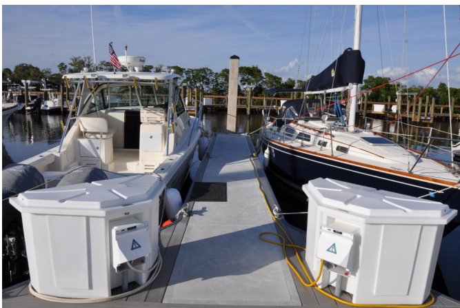
Concrete floating dock with power plugged into boats.
