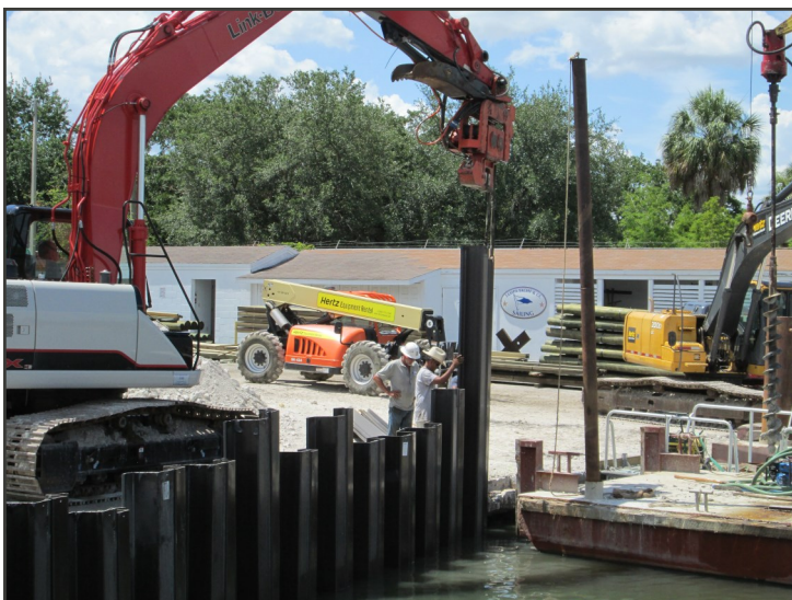
Installing new seawall panels outside of the old walls.
