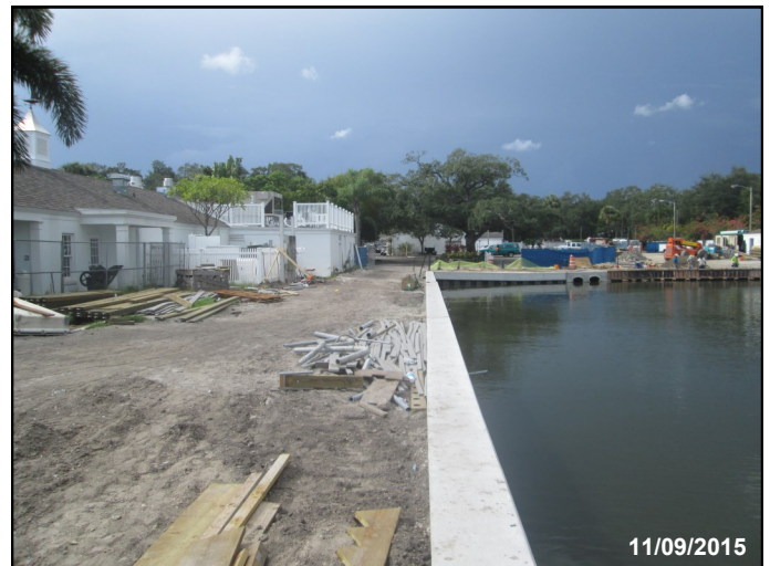
New seawall cap completed.
