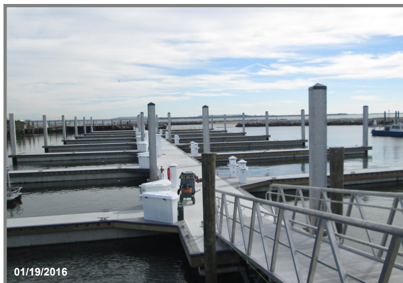
New concrete floating docks in place.
